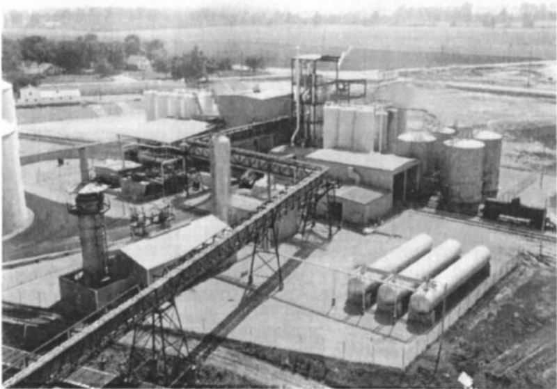
Figure 8. Typical bulk storage and handling facility for finished products.
